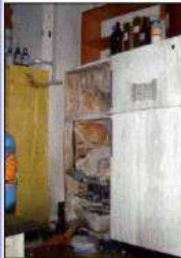
University of Virginia: A thermostat spark ignited flammable vapors.
